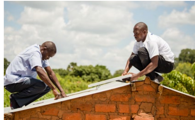
Solarworx employees install a rooftop solar panel.
