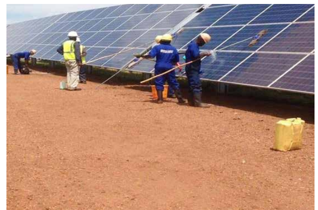
Figure 14: Washing of panels to improve efficiency [Courtesy Mr Chaim Motzen]
