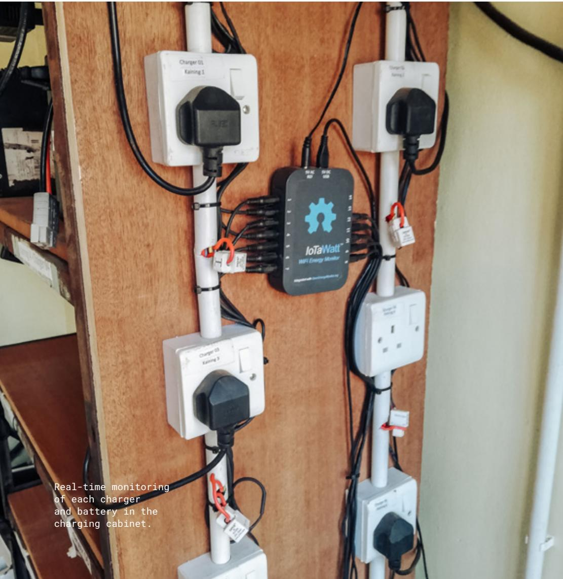
Real-time monitoring of each charger and battery in the charging cabinet.
